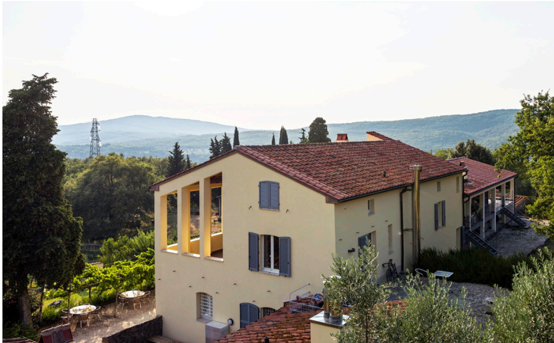
The view from southwest
